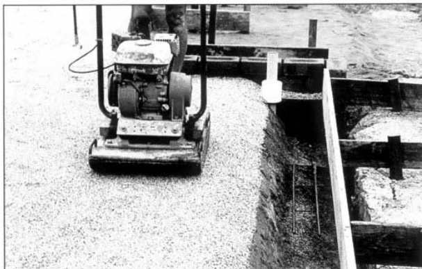
“GranitGard” – Being installed under a slab
