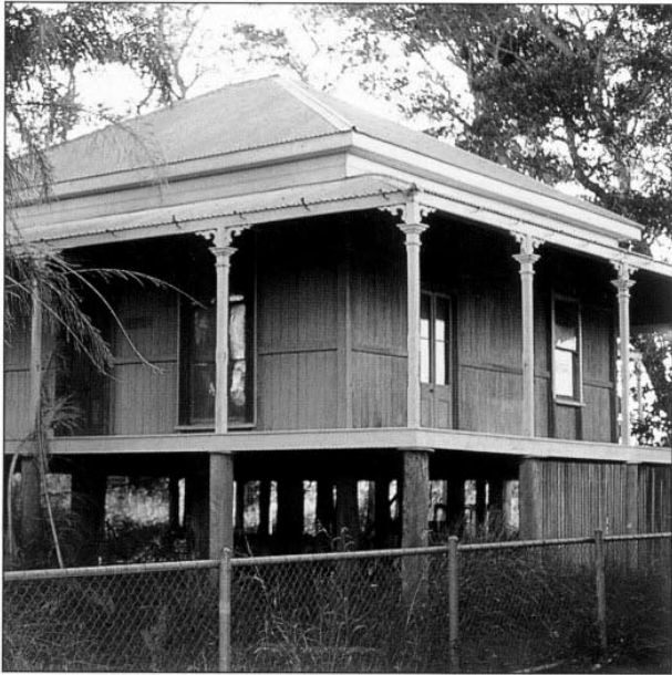
Traditional construction: For over 200 years ground separation has provided effective termite protection
