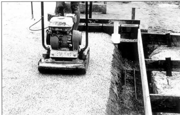
“GranitGard” – Being installed under a slab
