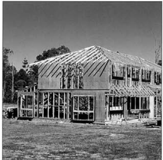
Slab-on-ground construction – Requires more permanent protection methods due to inaccessible areas such as under the slab
