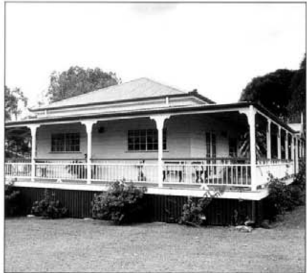
Suspended timber floors – Protection is easily provided by ant caps and regular inspection
