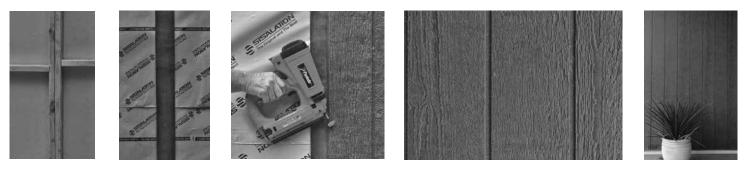
Fixings must be provided at 200mm centres to the studs and plates nearest the edge of the sheet, and 200mm centres throughout the centre of the sheet to all underlying studs and noggings. Fixing shall be no closer than 12mm from the sheet edges and must not be in the grooves of the sheets. Drive fixings flush with the sheet surface. No punching is permitted. Refer to the fixing details for pre-primed Weathergroove.
