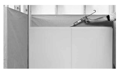
Position the first board of the below ensuring the Self-lockin second row of Rubix Panels w as per fixing instructions for th Repeat for the subsequent pa and sealing horizontally as at
