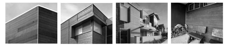
**Note:** Natural Products are composed of unsealed natural hardwood timber which may occasionally exhibit tannin bleeding. Consideration must be taken if installing unsealed Weathertex products above porous or light coloured features.
