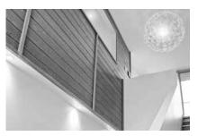
Butt joins may be lined up vertically on stud and capped by a (45mm min.) timber batten, 6mm minimum control gap, and Alcor back flashing with sealant
