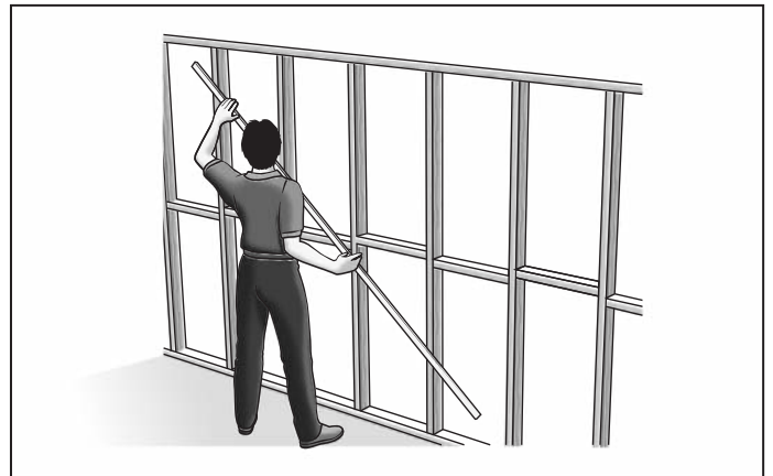
FIGURE 1 FRAME STRAIGHTNESS
