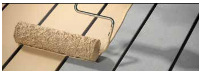
FIGURE 15 APPLY EXTERIOR TRAFFICABLE PAVING PAINT OR SEALER
