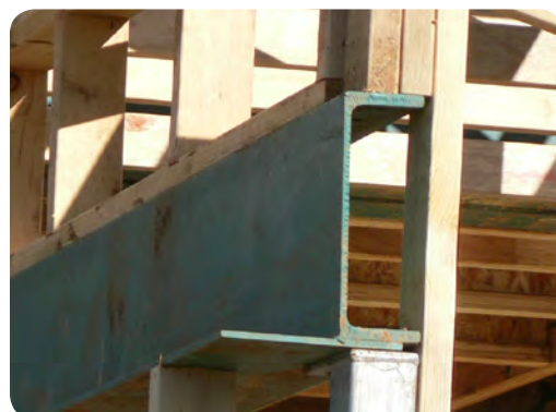
Figure 46: Thermal bridging.
