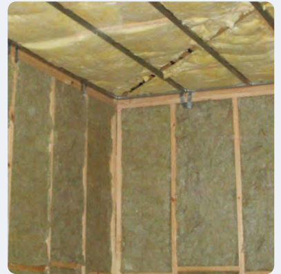
Glass-wool bulk insulation batts.
