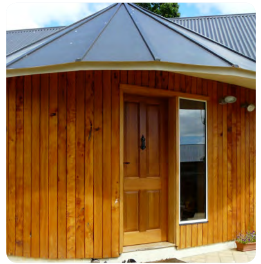
Figure 54: Traditional cladding over rigid board insulation. Timber ship-lapped boards over polystyrene board. Photo: Mark Dewsbury
