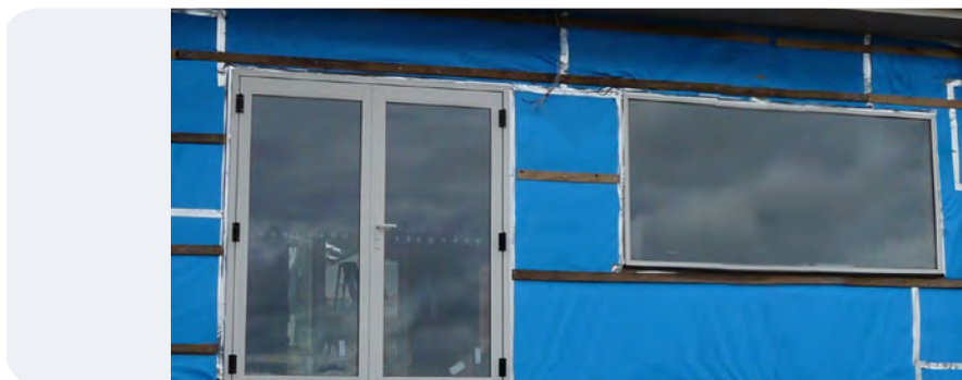
Figure 21: Tape joints. Building wrap covers all walls and is overlapped and taped. Photo: Mark Dewsbury
