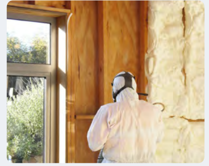
Sprayed-in-place wall insulation
