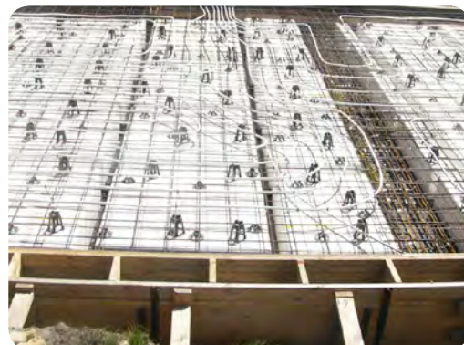
Figure 37: Underslab waffle-pods. Underslab insulation is suitable for cooler climates. Photo: Mark Dewsbury
