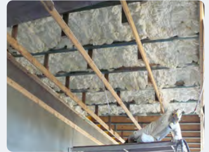
Sprayed-in-place wall insulation
