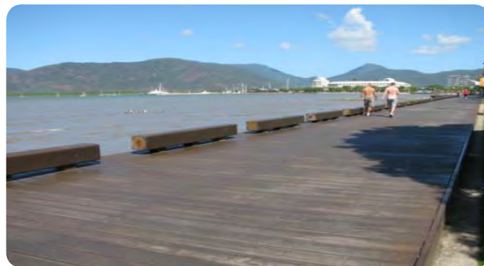
Figure 18: Site-applied pigmented deck stain requiring maintenance.
