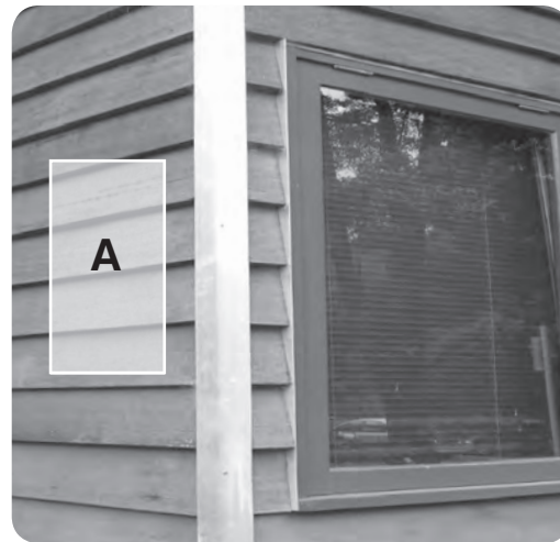
Figure 21: Detailing green timber weatherboards to allow movement.
