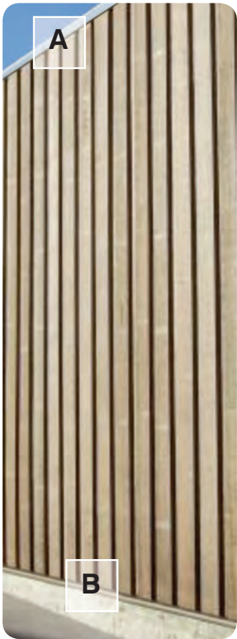
Figure 15: Detailing to avoid standing water.
