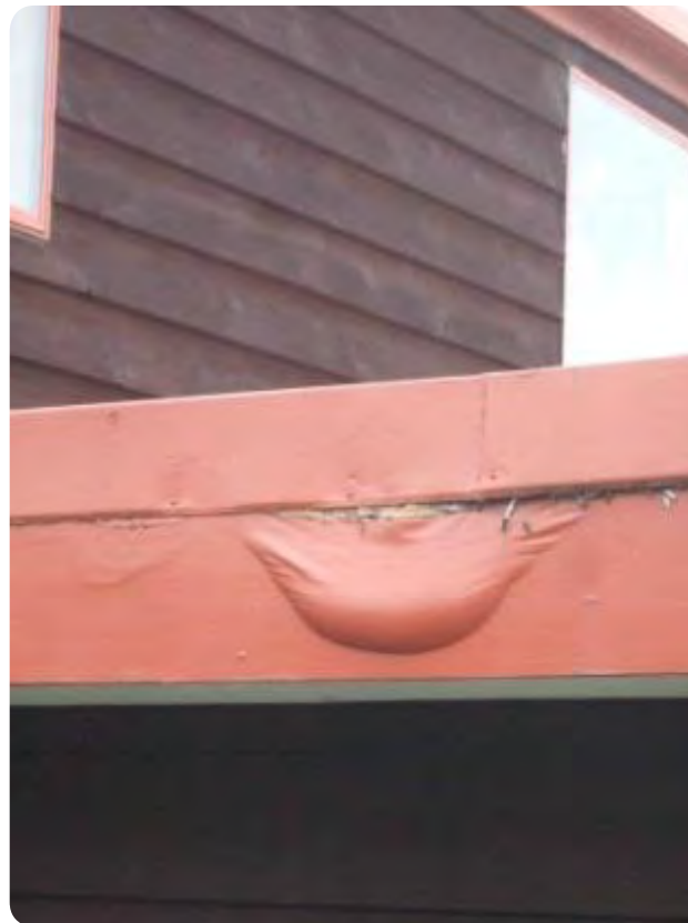
Figure 16: Poorly maintained paint which is trapping moisture.
