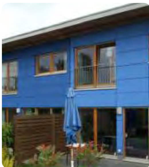
Figure 7: Painted plywood cladding, varnished timber joinery.
