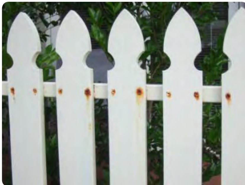
Figure 20: Rapid corrosion of poorly specified fasteners.
