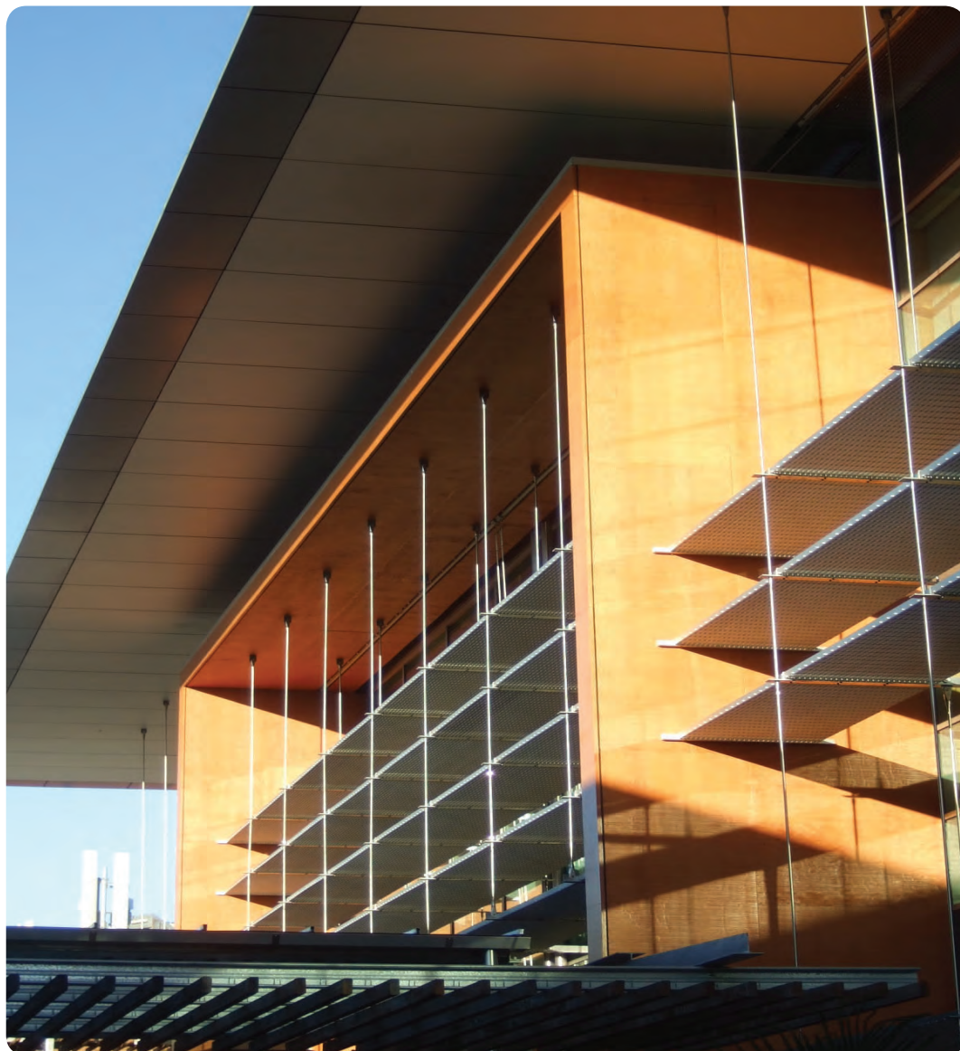
Figure 6: Stained and coated external plywood cladding.
