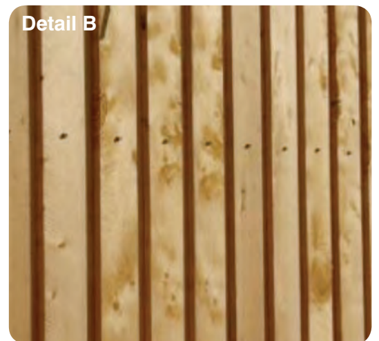
Figure 22: Visually significant fasteners; vertical green timber cladding.
