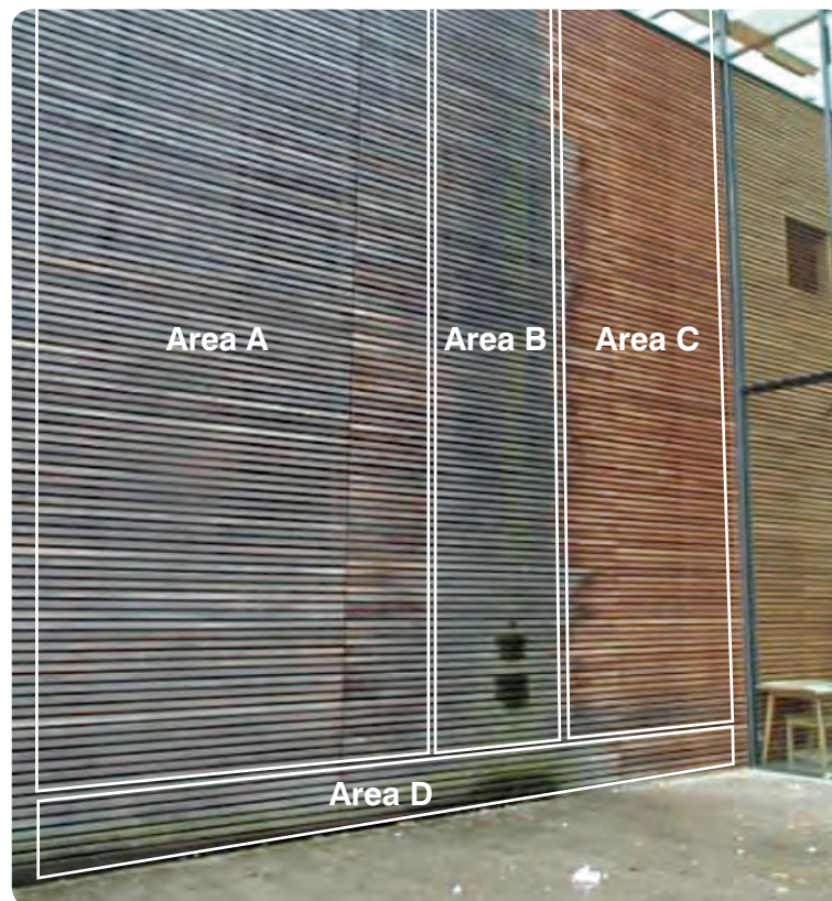
Figure 10: Differential weathering across a façade.
