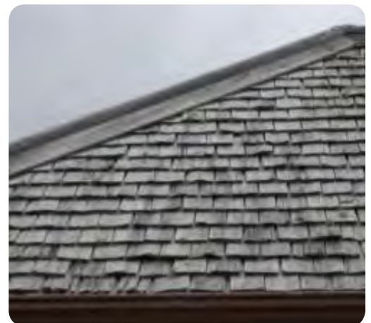
Figure 12: Bare timber shingles.
