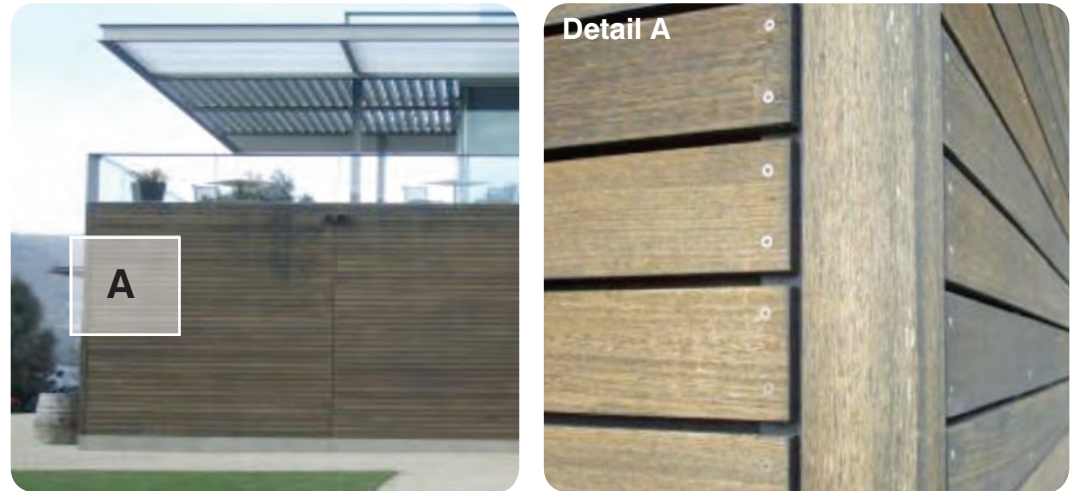
Figure 23: Visually significant fasteners, seasoned horizontal cladding.
