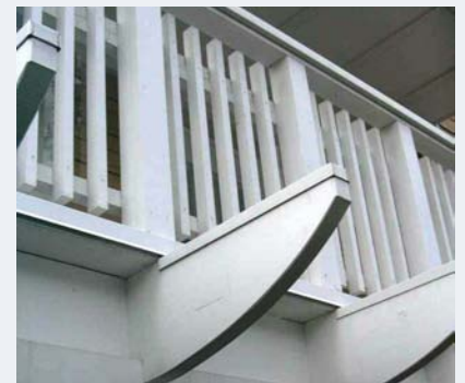
Capping protects top and end grain of projected beam.
