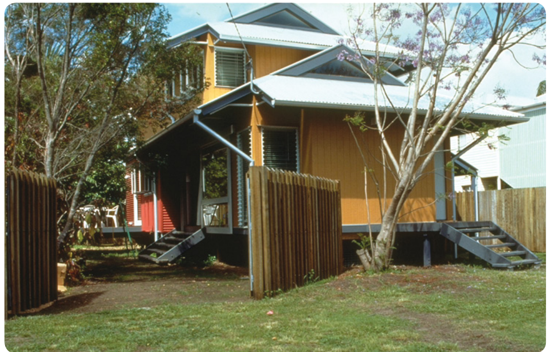
Large overhangs provide good protection.
