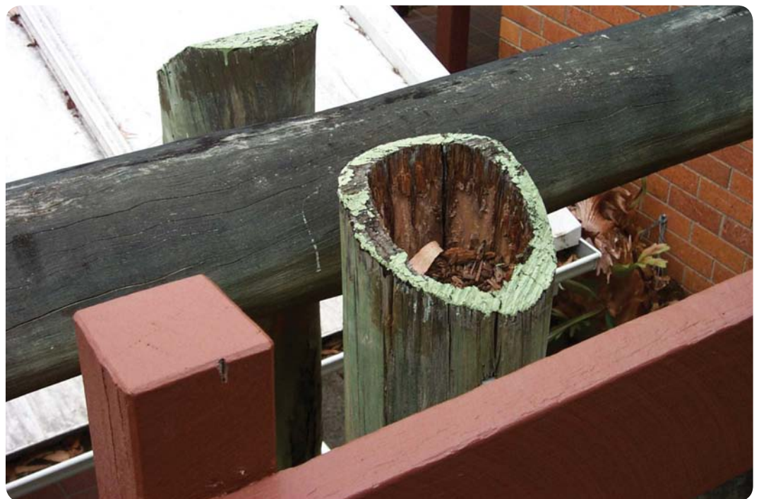
CCA treated sapwood outperforming durability class 2 heartwood
