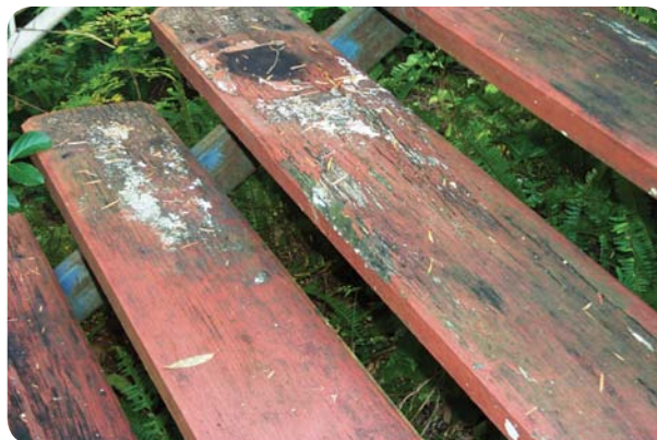
Poor maintenance of stair tread.
