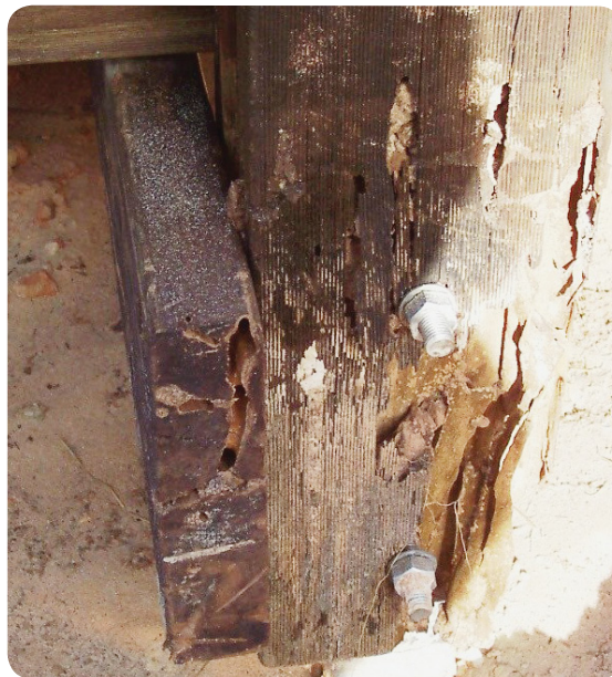
Termite damage to non-resistant timber.
