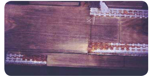
Corrosion of nail plates on deck joists after 6 years exposure near surf beach.
