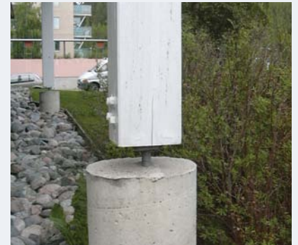
A well-ventilated, free-draining post support.
