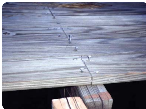
Plain shank decking nails in pine have ‘worked out’ with cyclic wetting and drying.
