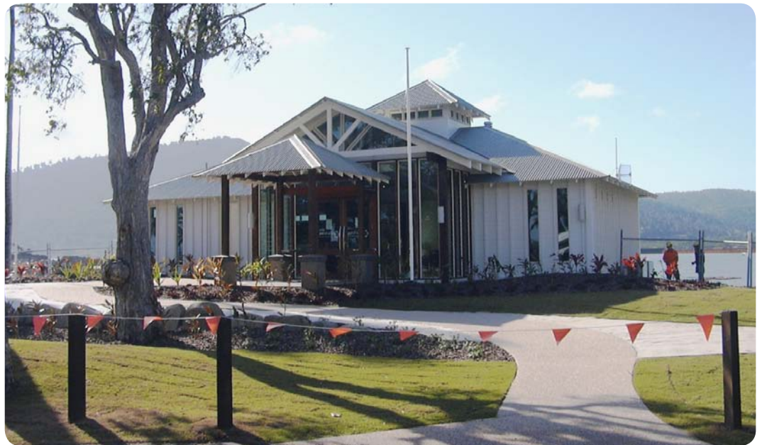
Roof overhangs provide good protection to timber walls below.
