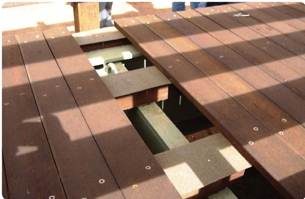
Good detailing (staggered screws and DPC over joists) used for this prefabricated bridge.
