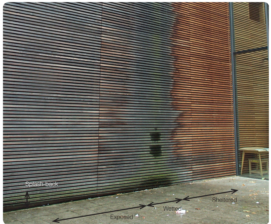
Figure 6: Differential weathering and decay on a facade.
