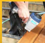
Position Gun Into Grooved Decking & Shoot !
