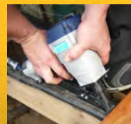
Position Gun Into Grooved Decking & Shoot !
