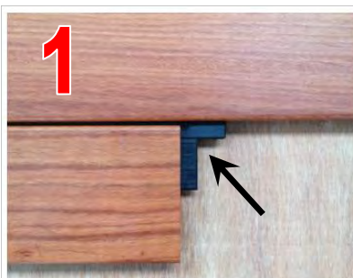
1/ Insert Rear Half of DeckBone
