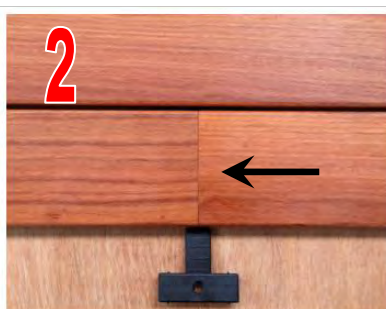
2/ Insert Next Decking Board
