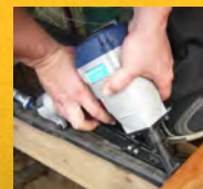
Position Gun Into Grooved Decking & Shoot !
