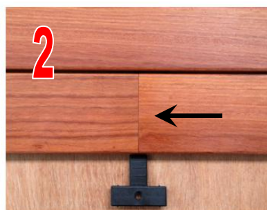
2/ Insert Next Decking Board
