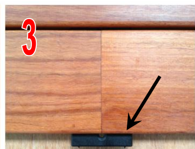
3/ Insert Front Half of DeckBone
