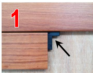
1/ Insert Rear Half of DeckBone
