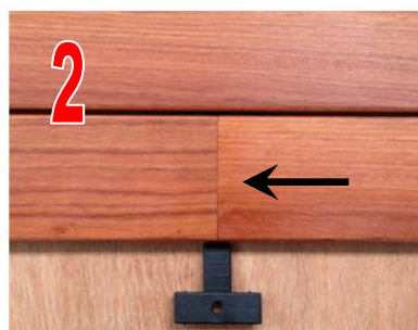
2/ Insert Next Decking Board
