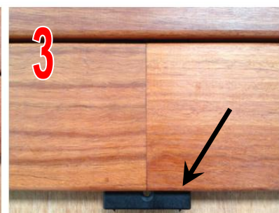
3/ Insert Front Half of DeckBone
