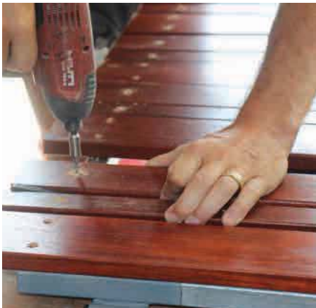
STEP 7. Fix your gate or panel cladding to your Quick Frame gate or panel.
