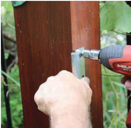
STEP 4. Hang your hinge receivers to post or wall.
