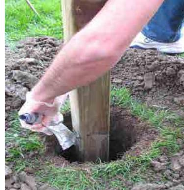
10. Adjust the post if necessary for up to 10 seconds. Do not move the post up and down. Expansion will finish in approximately 3-5 minutes and there will be no need to brace or hold the post after that (hold the post for 5 minutes in windy conditions). In approximately 15-30 minutes Fast 2K will already be quite hard. Wait for approximately 2 hours for the product to completely set before installing the fence or gate.
