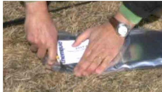
9. Empty the bag into the hole, "wetting the post" by pouring some of the composite on the post itself at ground level. Wetting the post helps to provide a good seal to the post.
