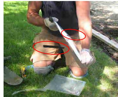
7. Rub the bag with force from top to bottom along any hard surface that has no sharp edges (for example rounded edge of a saw horse, a drill, a tool box or a table). Mix for 20 to 30 seconds by forcing material inside the bag from one end to the other with each stroke ("shoe shinning" technique). **DO NOT EXCEED MIXING TIME AS BAG MAY RUPTURE.** **NOTE: If the bag is above the recommended temperature before mixing – the product may expand too fast.**
