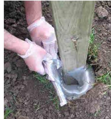
12. CLEAN UP: Using Chemque's Fast 2K<sup>TM</sup> Remover and a soft cloth, carefully remove any Fast 2K<sup>TM</sup> smudges from the post surface as well as tools and equipment **before Fast 2K<sup>TM</sup> dries**. After Fast 2K<sup>TM</sup> dries, it can only be removed mechanically with a shovel, sand paper or a utility knife which may damage the post.
